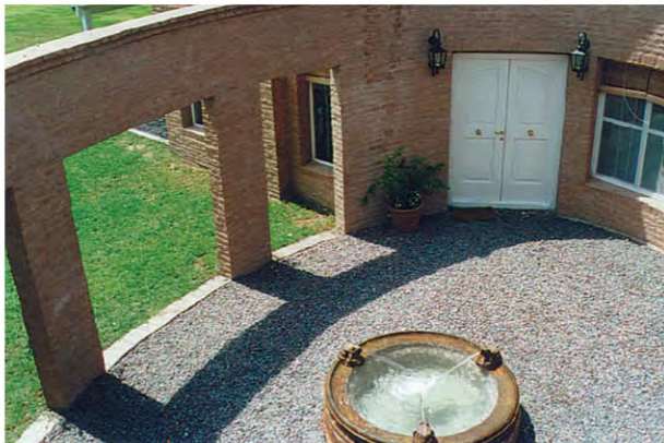
Court view Vista patio
