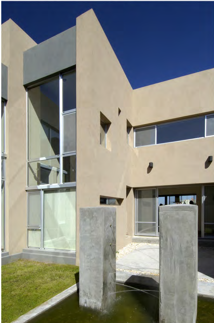
Court view Vista patio
